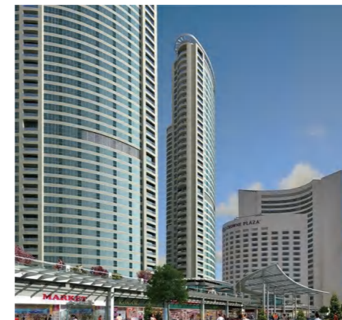
Umraniye & Esenler Tax Building, Turkey Calcium sulphate panel(homogeneous vinyl), 12,000m 2
